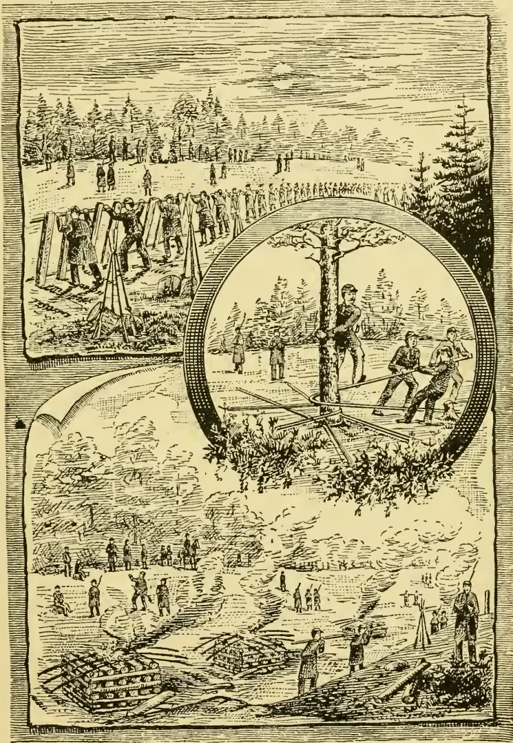
TEARING UP THE WELDON RAILROAD.
